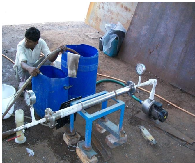
Fig 4: Setup of UF batch scale plant at Aastropure (P) Ltd
