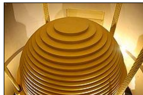
Fig 2(d): Tuned mass damper atop Taipei 101
