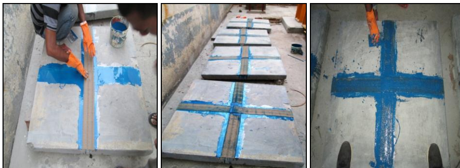
Fig 2: a) & b) Application of PPFRR, c) Retrofitted slab with PPFRR
